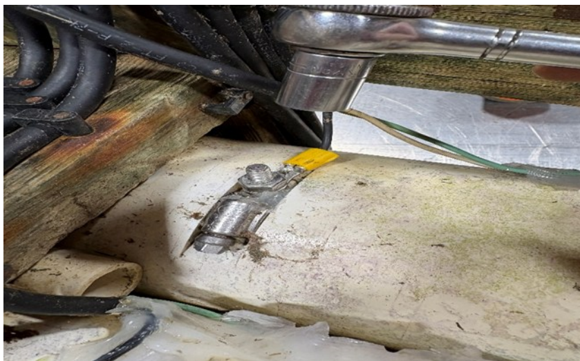
Figure C.7. A hose clamp with bolt for connecting the junction box wires to one of the tubes. The yellow ring terminal is where the wiring is attached, and the tube can be tightened typically with a 10 mm socket. .
