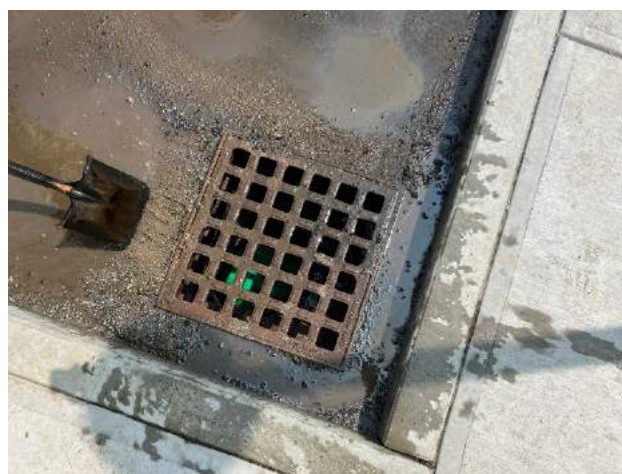
Remove debris and sediment from trench drains and catch basins.
