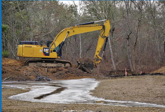
January 2021 – Dam Removal
