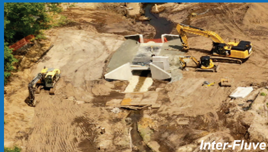
June 2021 – Construction of New Road
