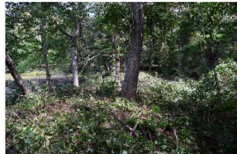
At right, view of the top of the earthen (primary) dam, looking east.
