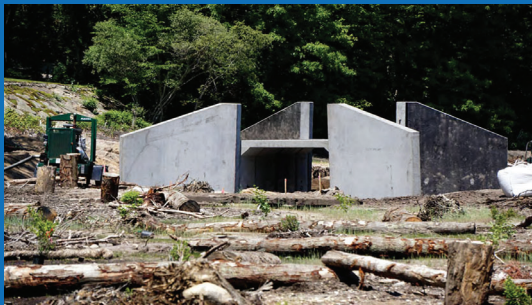
June 2021 – New Culvert in Place
