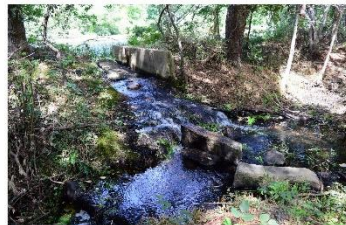
Downstream side of the dam's concrete spillway channel, view northwest.
