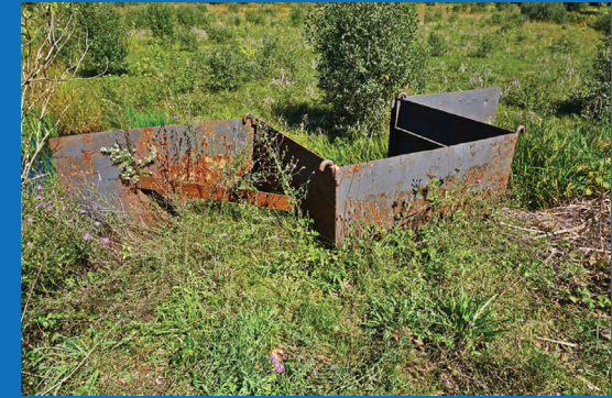
September 2018 – Bog Water Control Device Blocking Fish Passage
