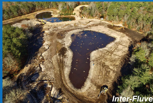
November 2020 – Ponds Completed
