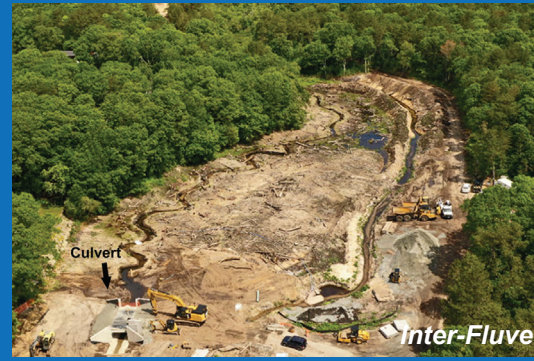
June 2021 – Culvert in Place
