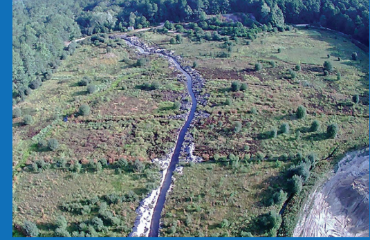
September 2020 – Diversion Channel
