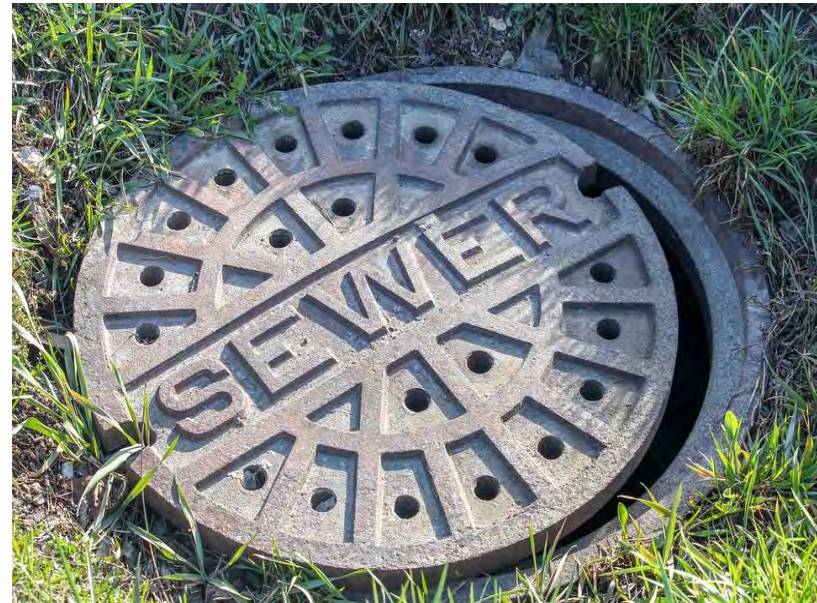
Figure 30. Sewer manhole cover (Pixabay).
