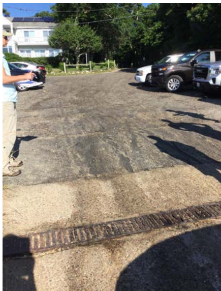
Photo Caption: Clogged trench drain at boat ramp
