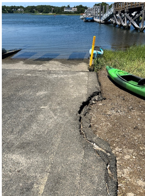
Photo Caption: Erosion and damage to boat ramp
