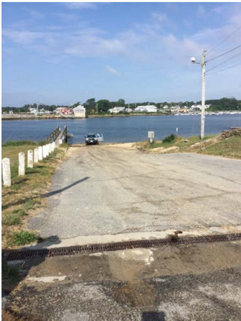
Photo Caption: Boat ramp with dock on the left and the clogged trench drain in the foreground.
