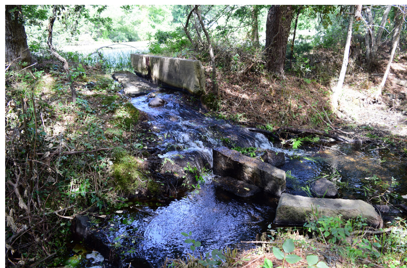
Downstream side of the dam's concrete spillway channel, view northwest.
