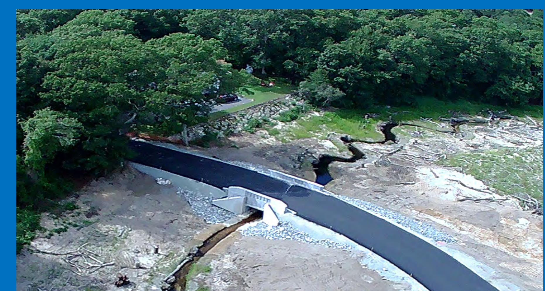
August 2021 – Road Paved
