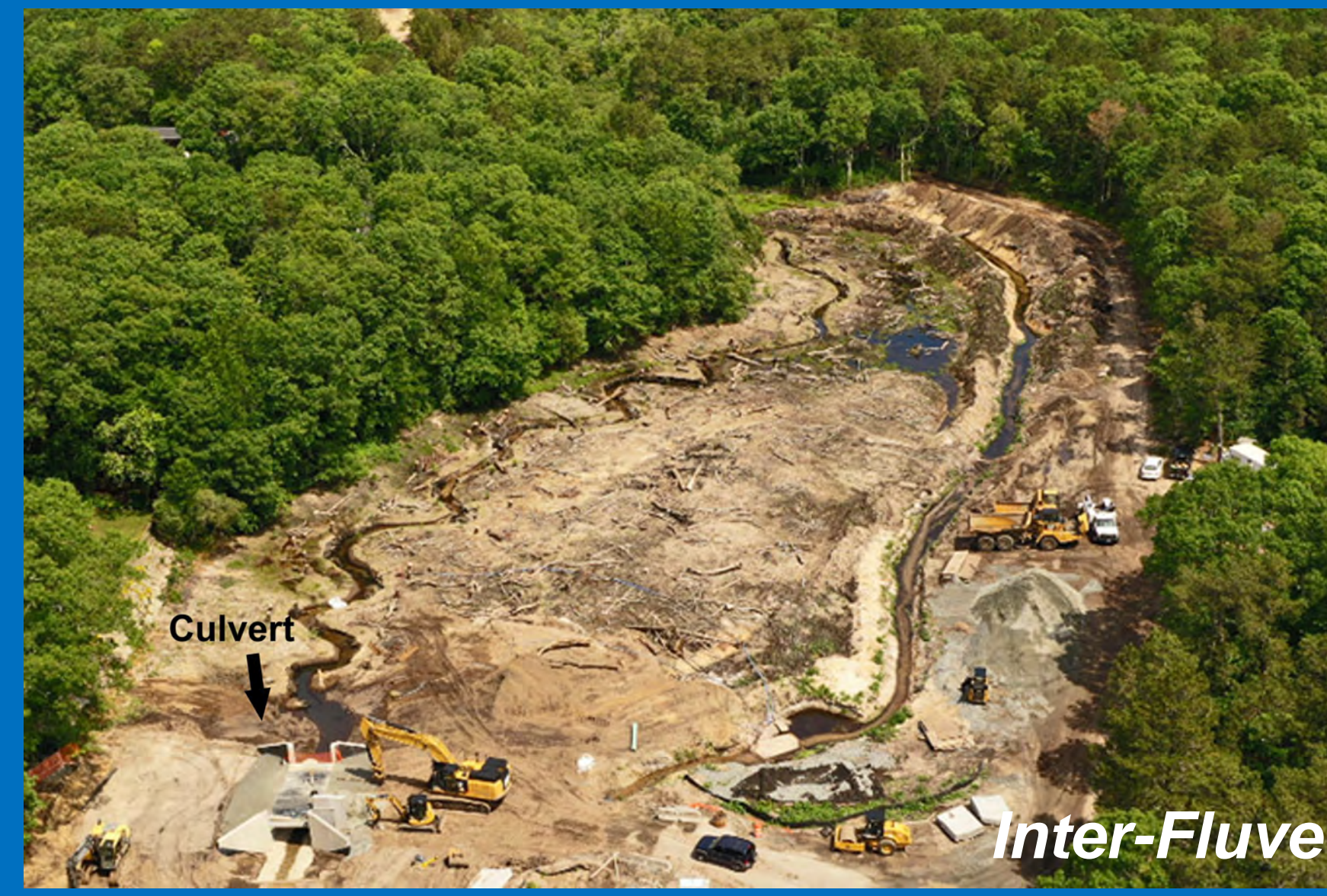
June 2021 – Culvert in Place
