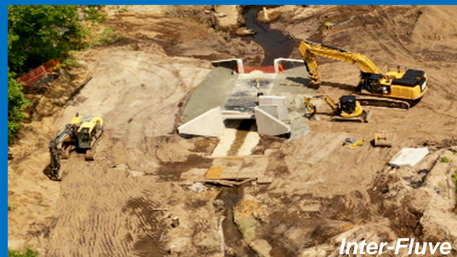
June 2021 – Construction of New Road
