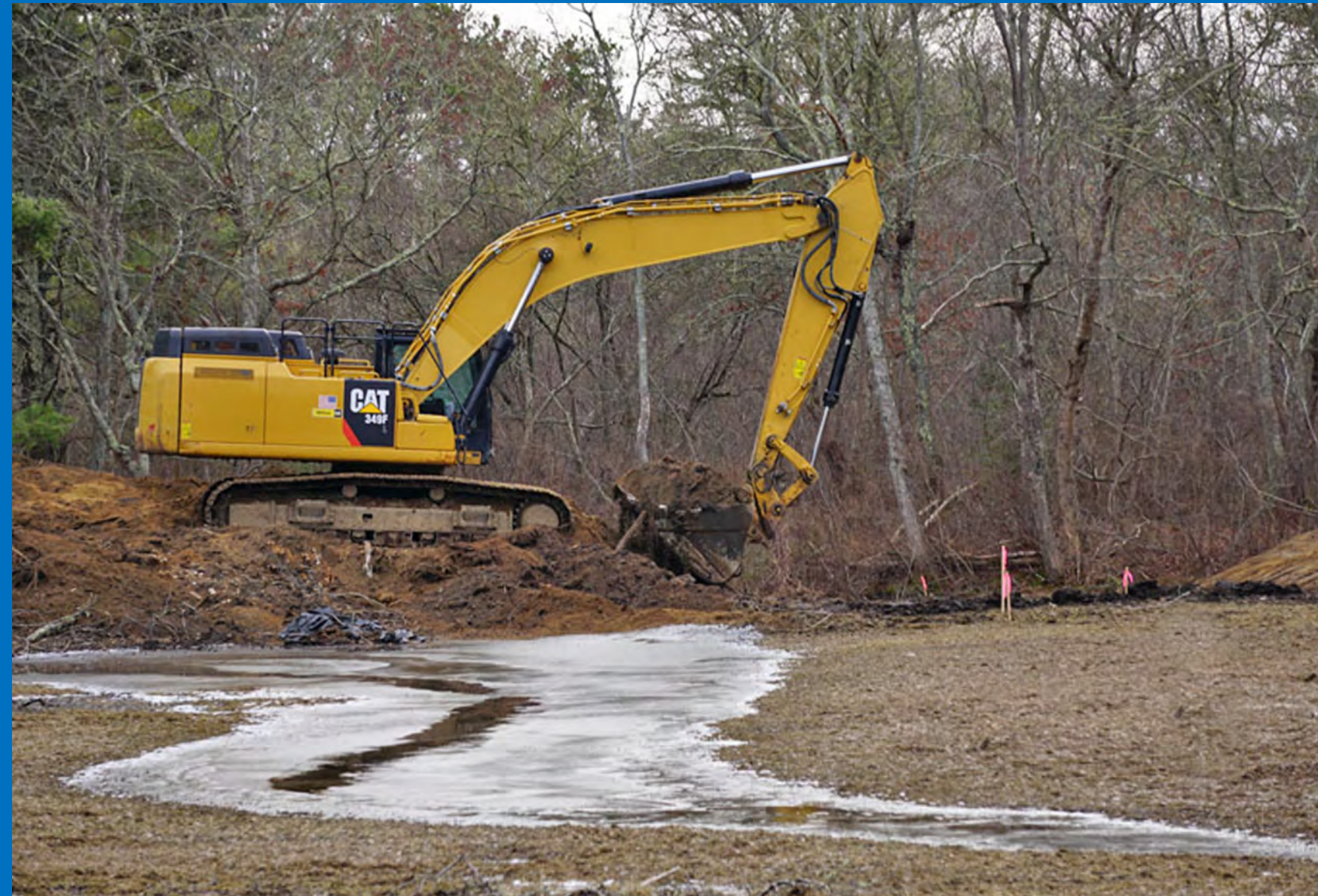
January 2021 – Dam Removal
