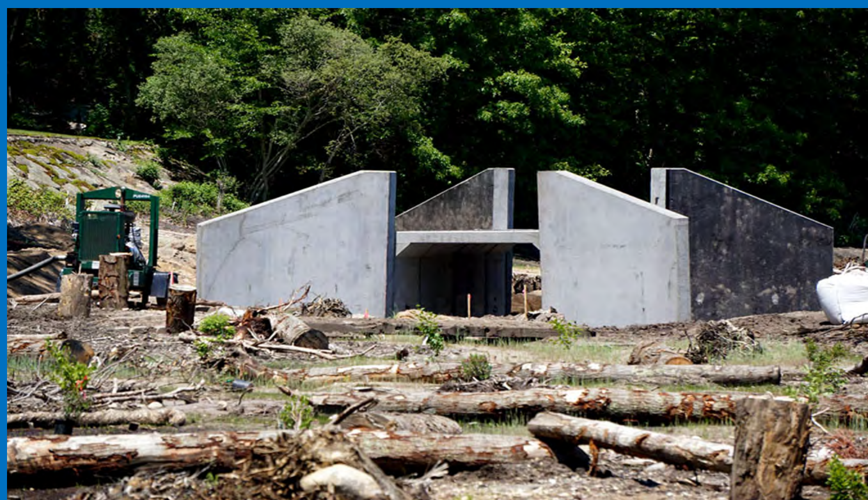
June 2021 – New Culvert in Place
