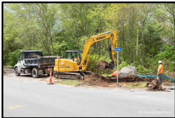
A smaller bioretention garden was installed along with the swale at the next intersection to treat additional runoff entering the river at this location.
