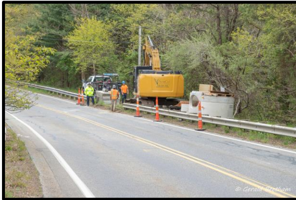
A water quality unit was installed in 2020 to remove sediment, trash, and other debris from road runoff before discharging to the stream.
