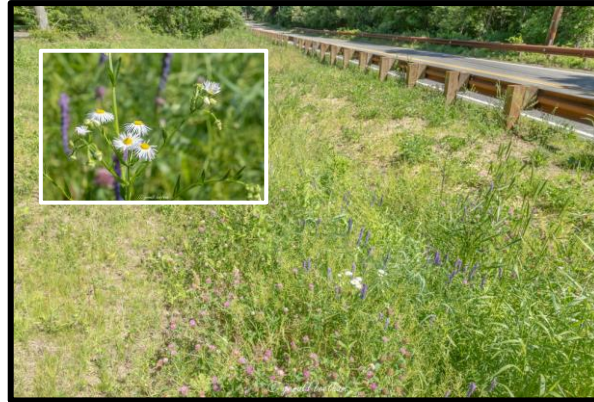
Designed for low maintenance mowing, this swale was planted primarily with grasses and was showing off its colorful blooms one year later.
