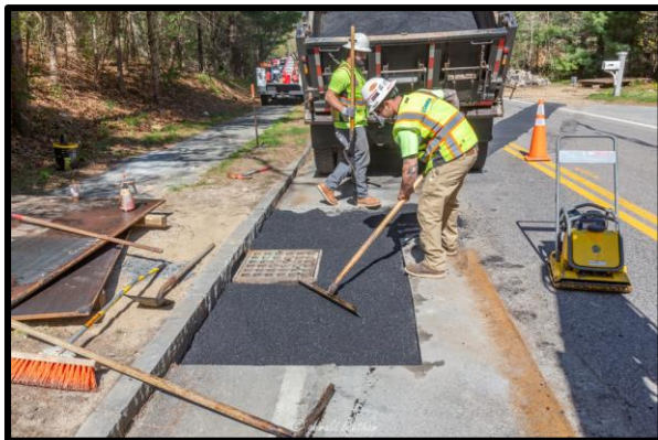
Additional stormwater runoff was directed into the swales through connection to existing catch basins across the road.
