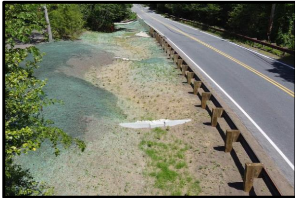
In 2020, a dry swale was installed along Putnam Avenue to address road runoff flowing into Little River and Cotuit Bay.
