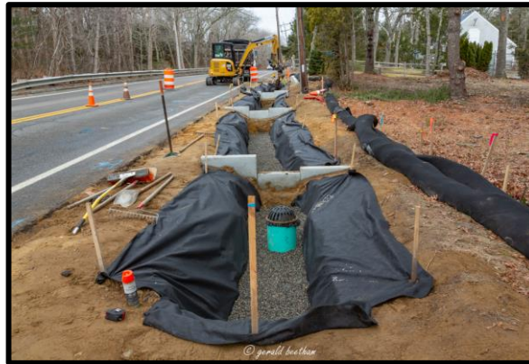
Two dry swales with a series of check dams and basins designed for the slope of the land were constructed in 2021.
