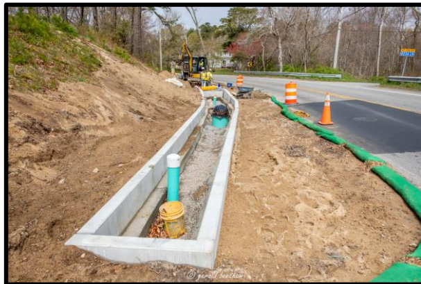
Concrete curbing lines both sides of the swales, an innovative design component to fit within the limited space between the hill and underground utilities.
