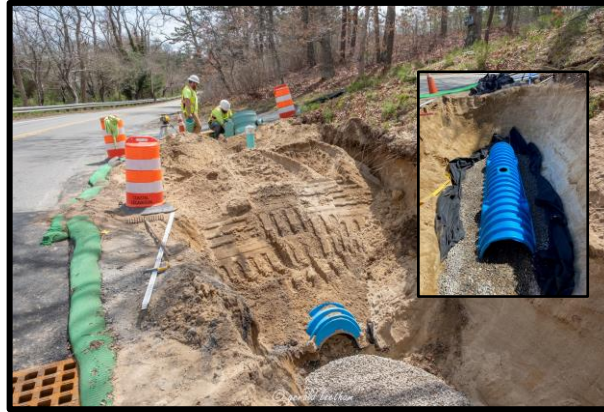
An infiltration basin was installed along with the swales to provide additional treatment and a new manhole installed in the roadway to connect to existing stormwater infrastructure (see inset photo to the right).
