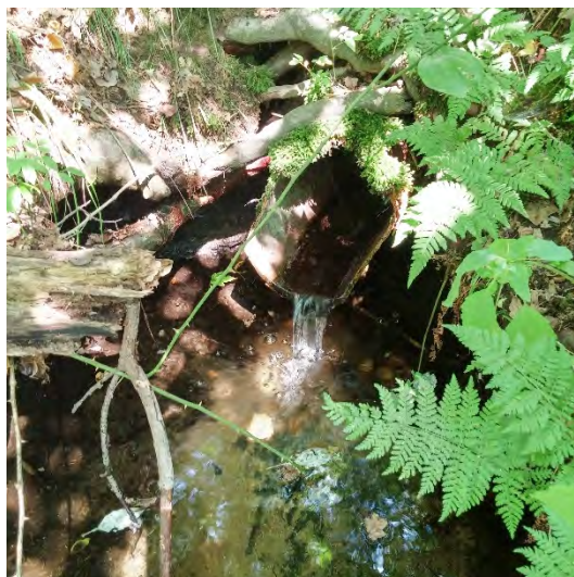
Photo 10. Small culvert running under Honey Suckle Lane in Chatham, MA that drains freshwater from the upper part of the watershed.
