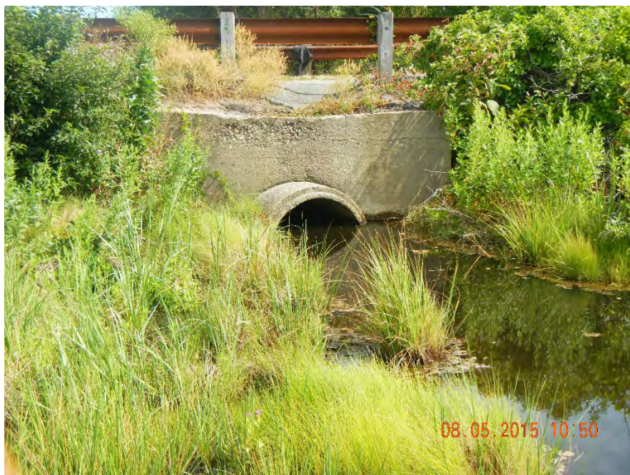
Photo 13. Park Avenue culvert on the seaward side of the marsh which is set in a concrete headwall (Yarmouth, MA).
