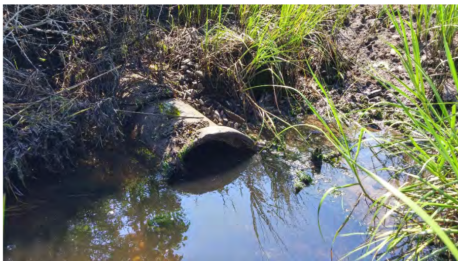
Photo 8. Restricted culvert running under Stage Harbor Road, Chatham, MA. This image was taken on the restricted side of the salt marsh.
