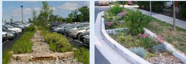
**Proprietary biofiltration systems** that incorporate plants and soils to capture and filter out pollutants.
