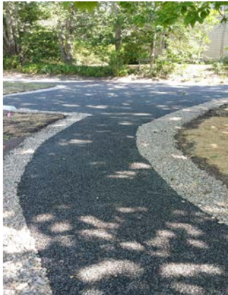
APCC believes that this may be the first installation of Porous Pave® for parking and path on the Cape.
